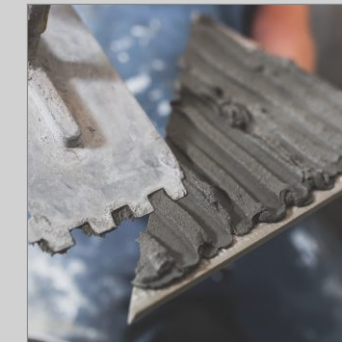
Cement Laying On Tile
