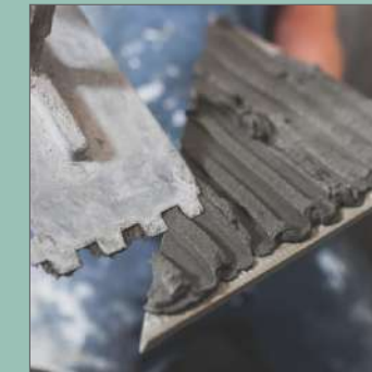
Cement Laying On Tile
