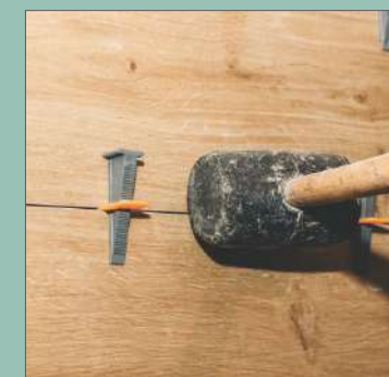
Remove Wedges Once It Dry
